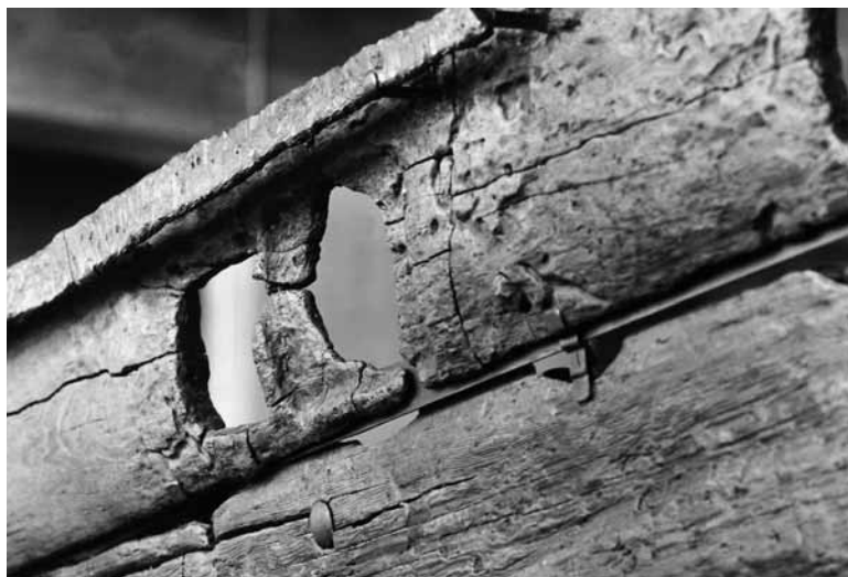
Fig. 26. Skuldelev 5. The shield-rack in position along the upper edge of the sheerstrake.
