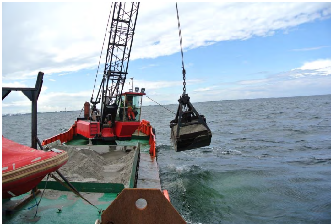
Figure 58: Sand is deposited from the vessel M/V Merete Chris onto the wreck.
